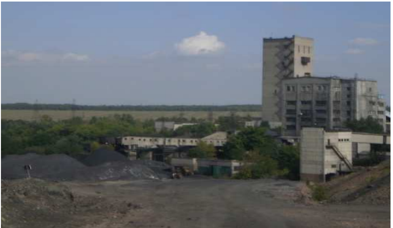
Figure 3 – General view of the concentrating mill
