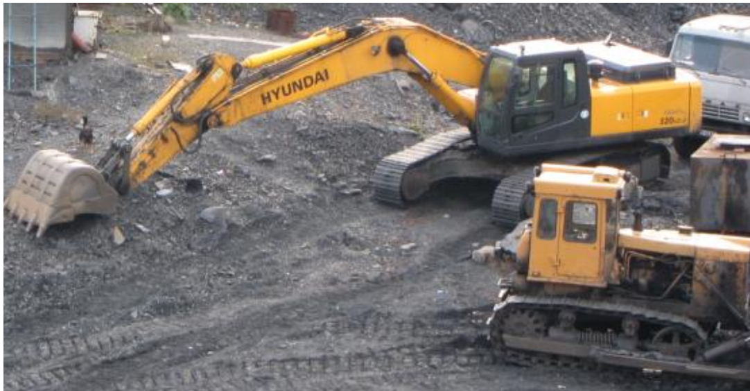
Figure 4 - Machinery involved in the project.
