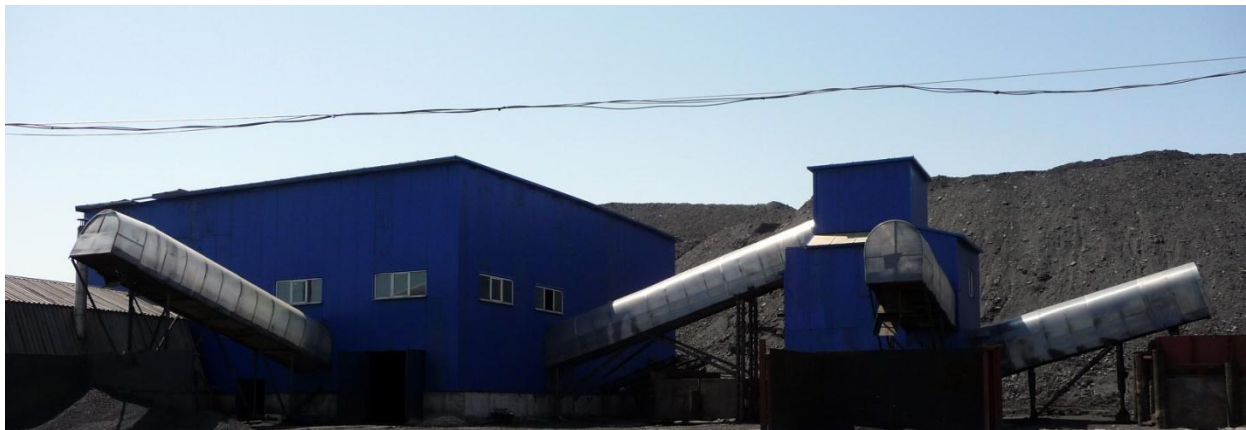
Figure 1 Project activity equipment
