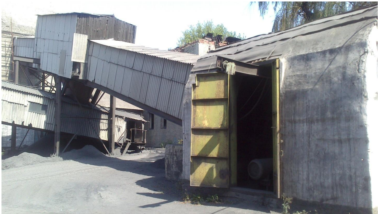
Figure 4 – Enrichment plant # 105 involved in the project.
