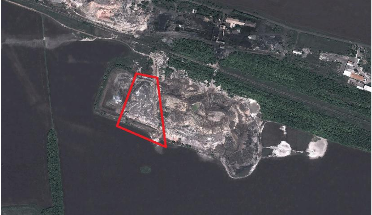
Figure 2 – Location of the waste heap # 8 at Kurahivska mine, view from satellite.
