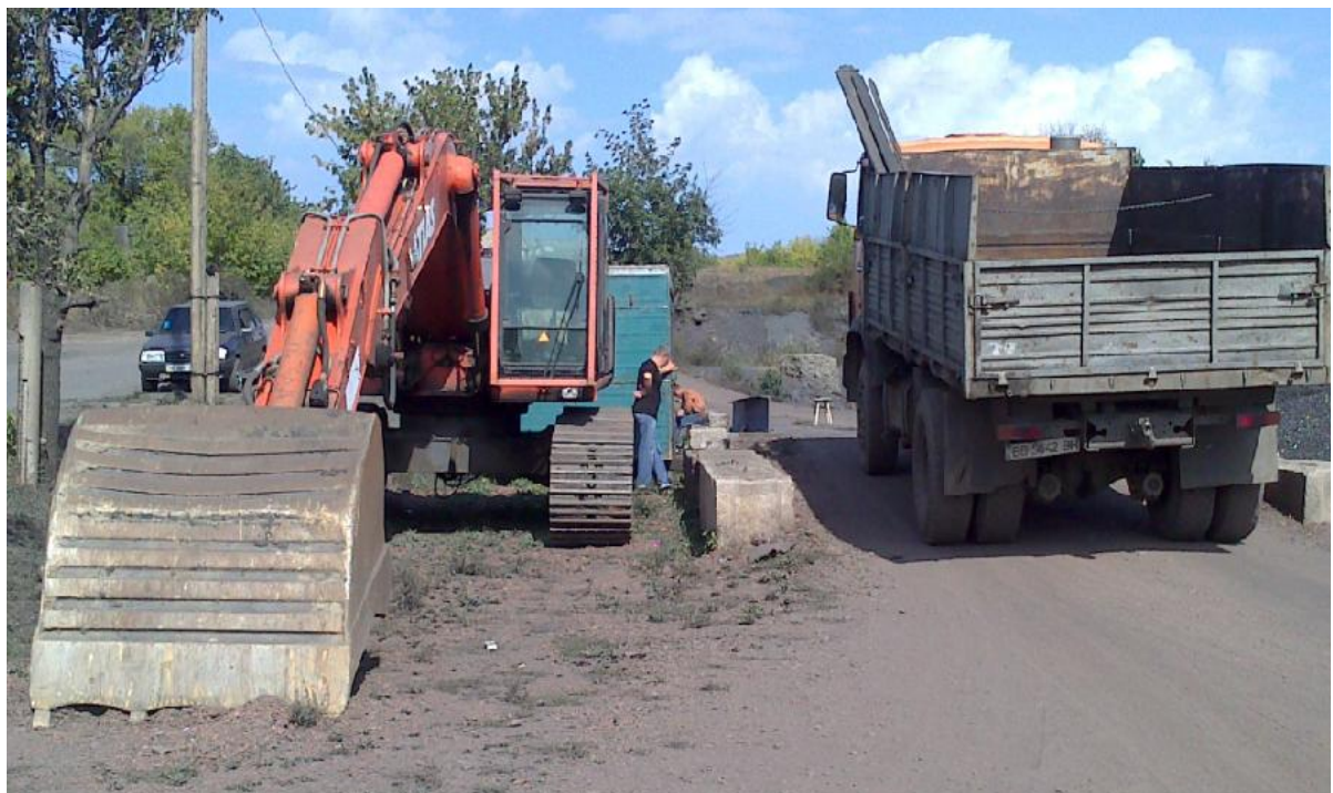
Figure 4 - Machinery involved in the project
