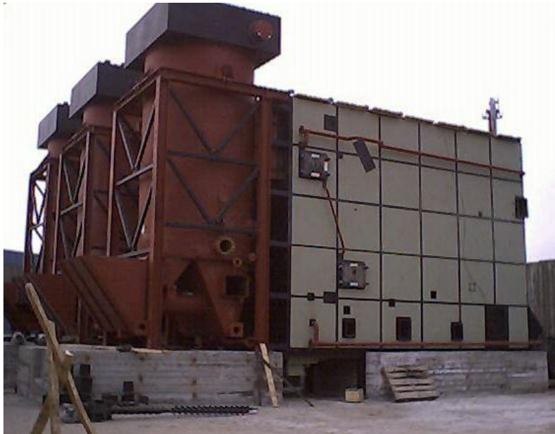
Fig. A.4-3. URBAS boilers during the boiler house installation phase
