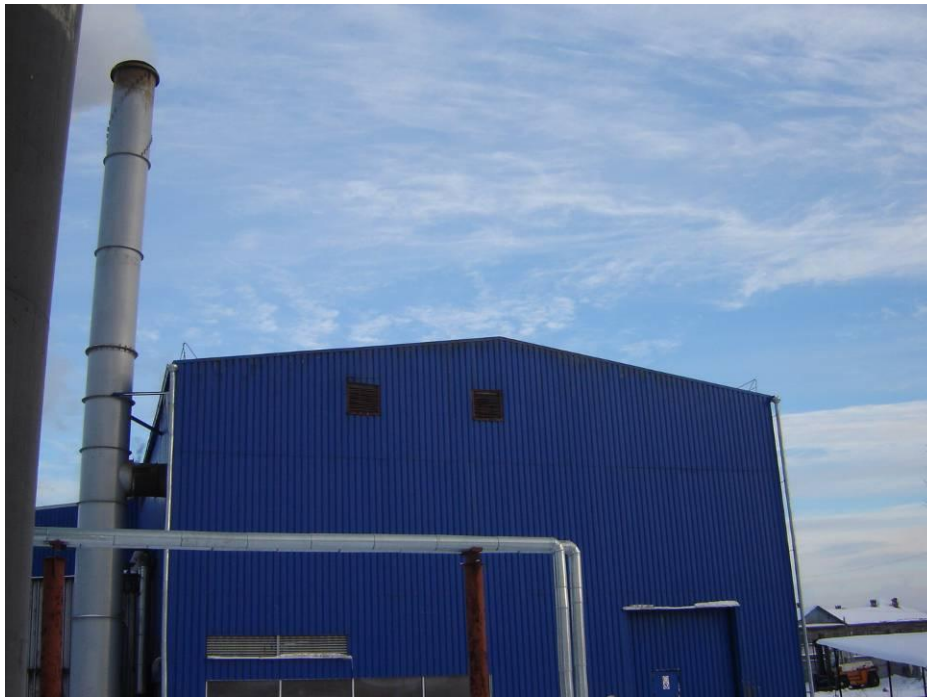
Fig. A.4-4. The new commissioned biofuel boiler house
