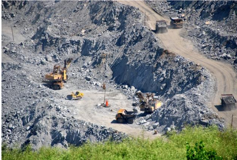
Figure 8 Works at Helyuvatskyi open pit.
