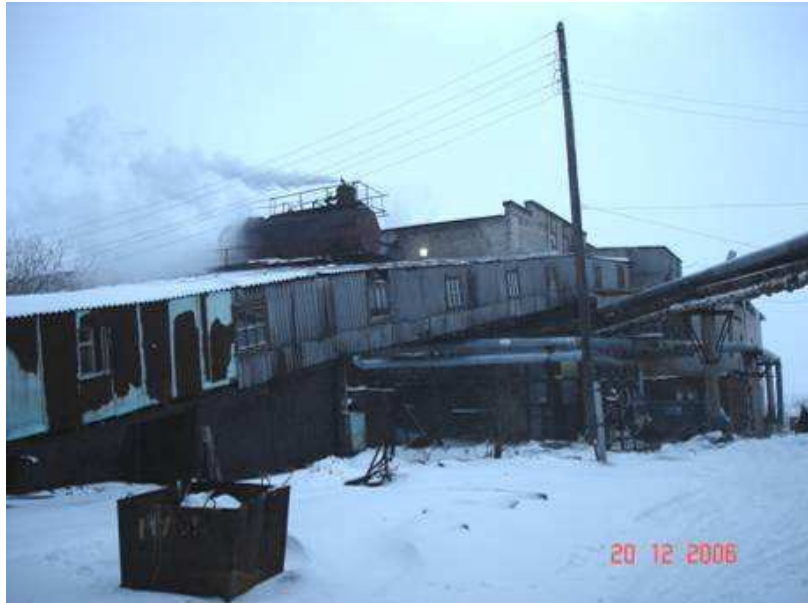
Fig. A.4-9. The old boiler-house at the Maimaksa production site
