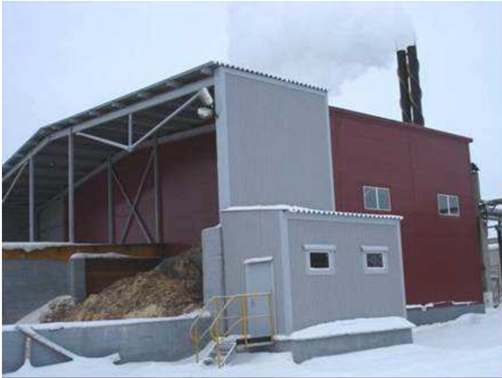
Fig. A.4-5. The new BWW boiler-house at the Tsiglomen production site
