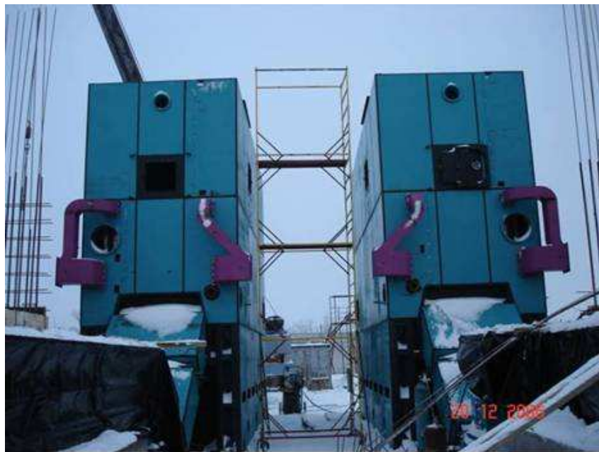
Fig. A.4-10. Construction of the new BWW CHP plant
