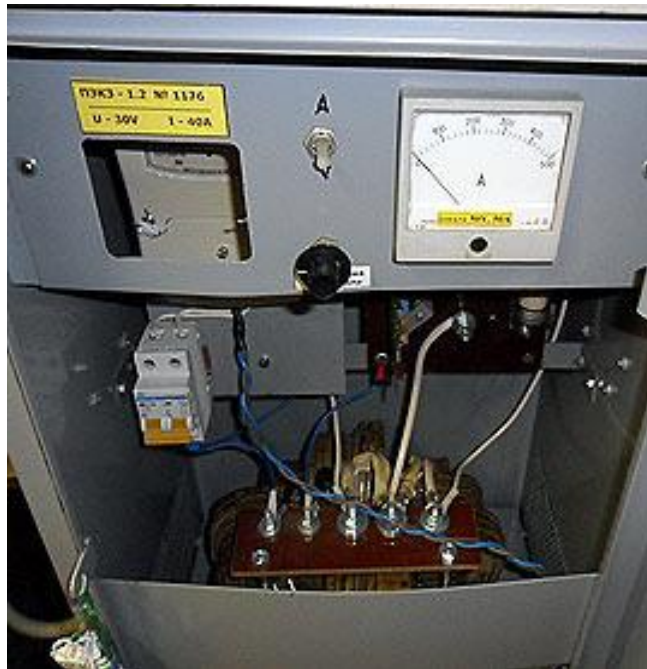
Figure 9. Cathodic protection electric transducer (CPET), produced by “Elkon”.
