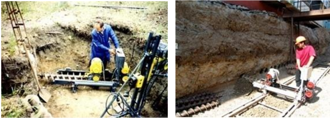
Figure 6. Operation of horizontal drilling machine
