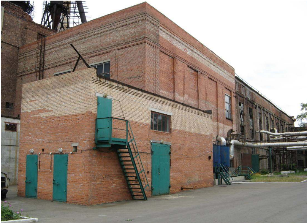
Figure 5. Place for extension of CHP as a result of the first stage of the project implementation
