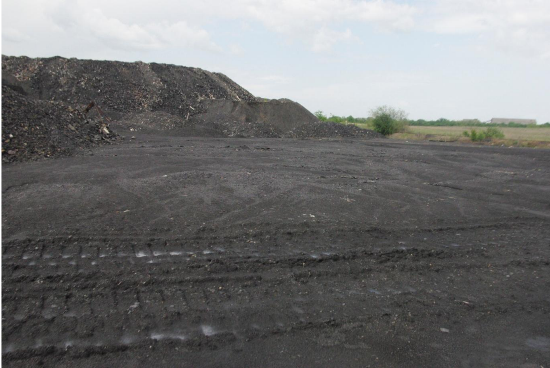
Figure 2 - The exterior of the waste heap under stage of dismantling
