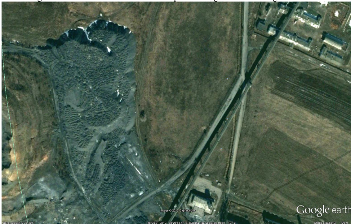
Figure 3 – The waste heap under dismantling, the appearance from the satellite
