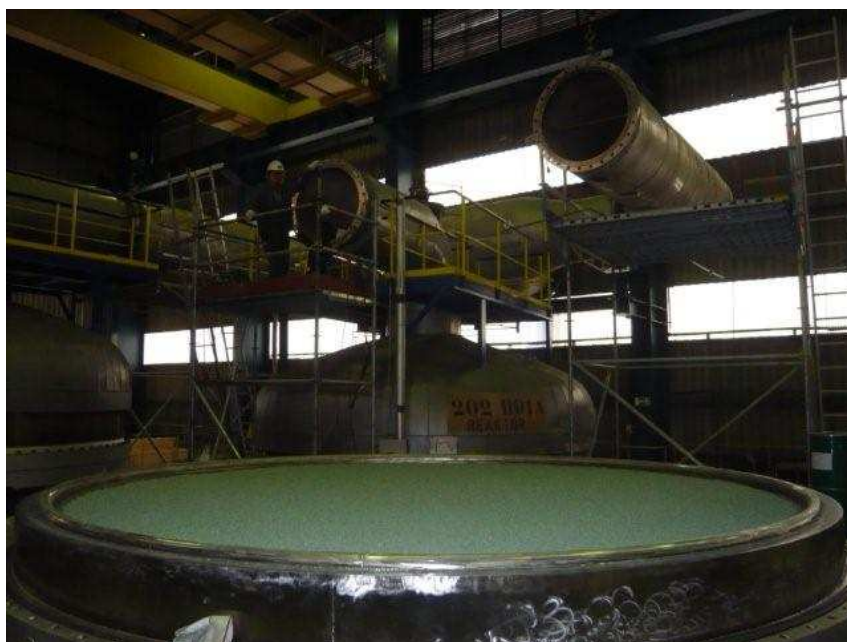
Figure 2: Installation of secondary catalyst
