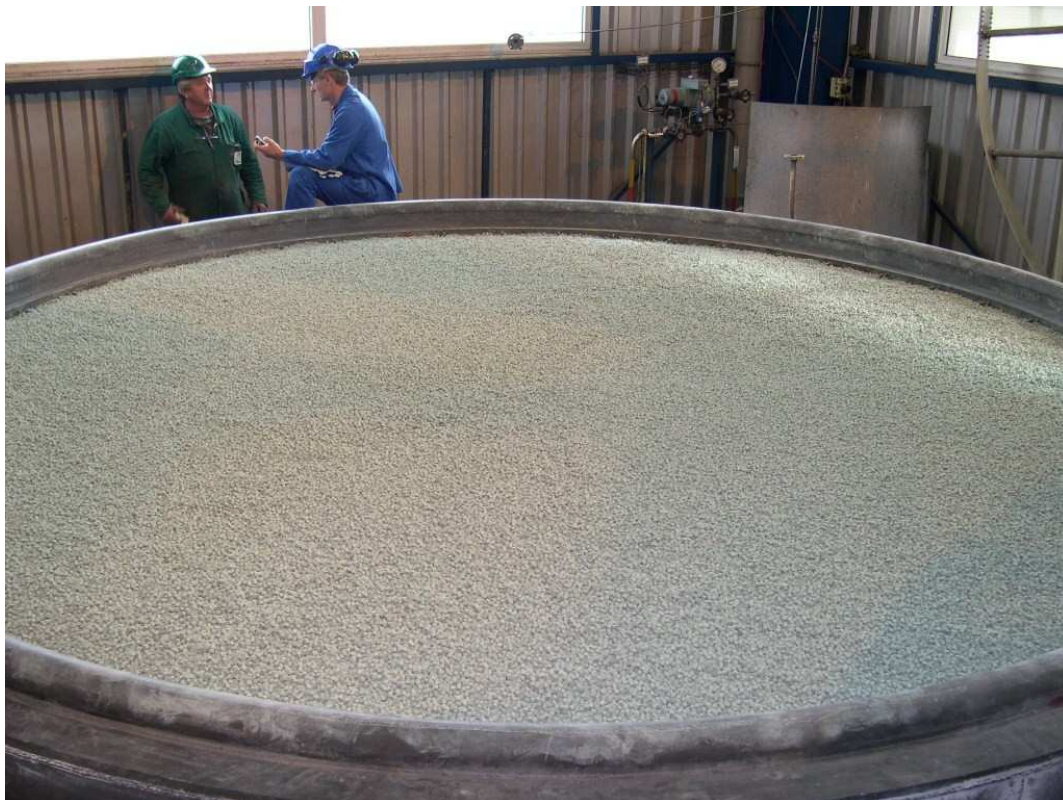
Figure 2: Installation of secondary catalyst
