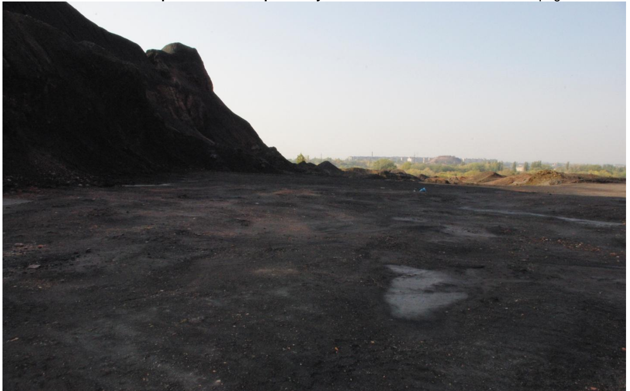
Figure 3 - The exterior of waste heap under dismantling stage
