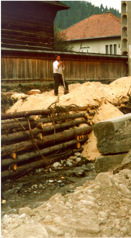
Fig: 2: Sawdust used for road construction
