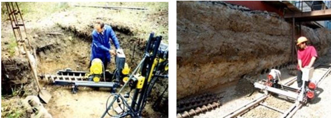
Figure 4. Operation of horizontal drilling machine
