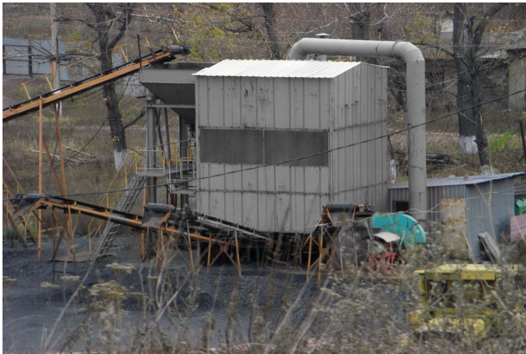
Figure 4: View of installation with a heavy environment for concentrating carbonaceous mass
