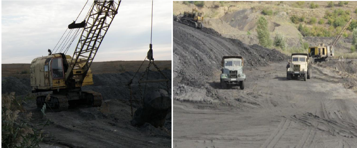
Figure 5 – Machinery involved in the project
