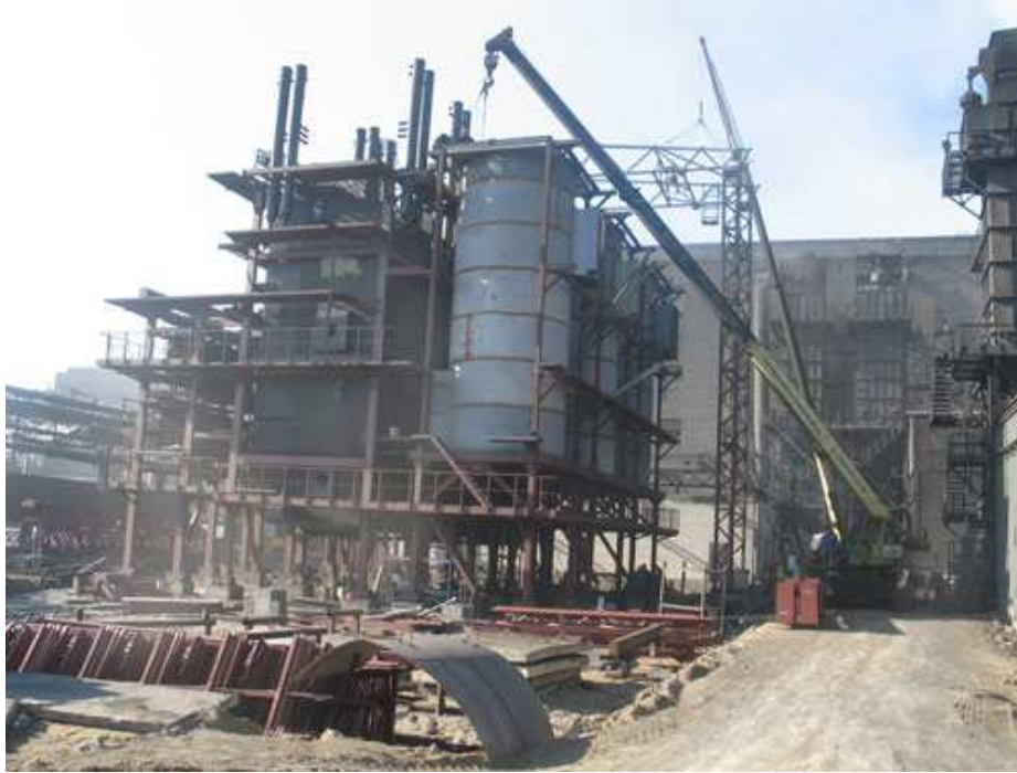
Fig.A-9. Exhaust boilers construction.
