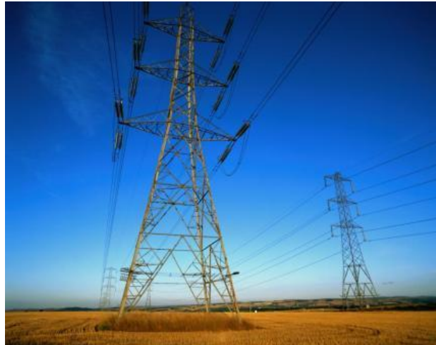
Figure 8. Towers of overhead power lines
