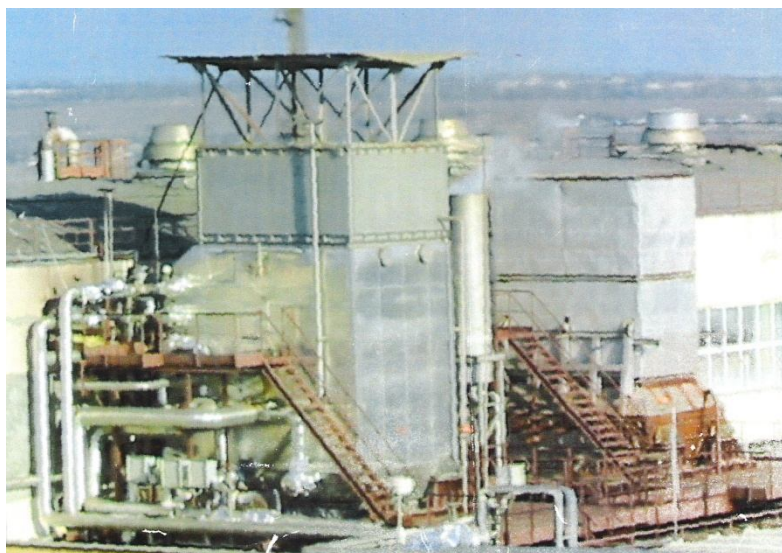
Figures 3 – a KUP-2500M waste heat boiler
