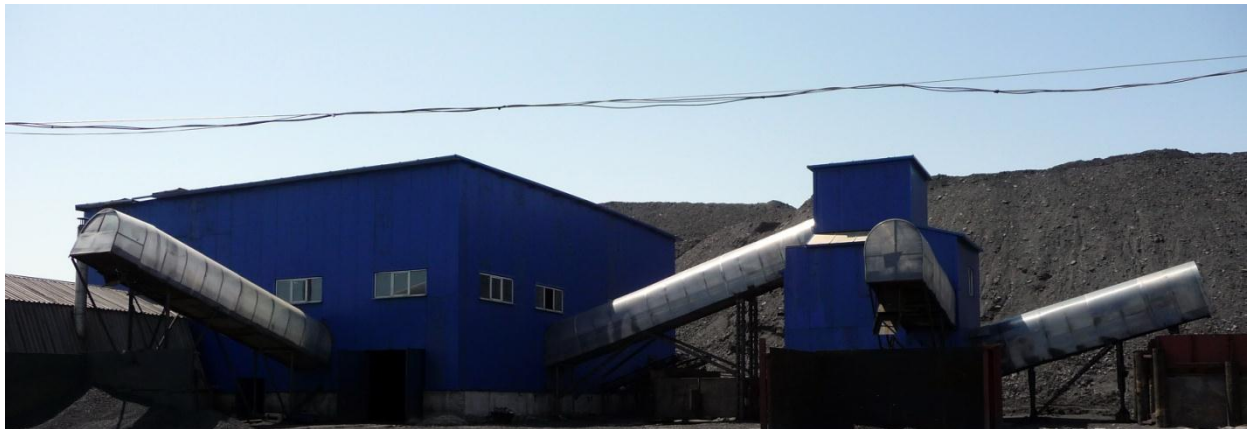
Figure 1 Project activity equipment
