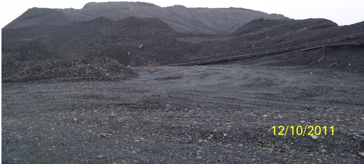
Figure 2 - The exterior of the waste heap of former mine "Rozsypnyanska-1" under stage of dismantling
