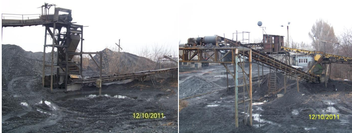
Figure 4 - Machinery for sorting rock mass
