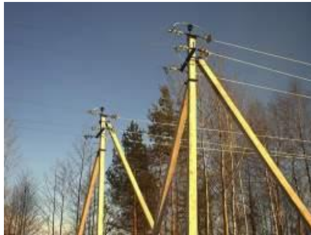
Figure 8. Towers of overhead power lines
