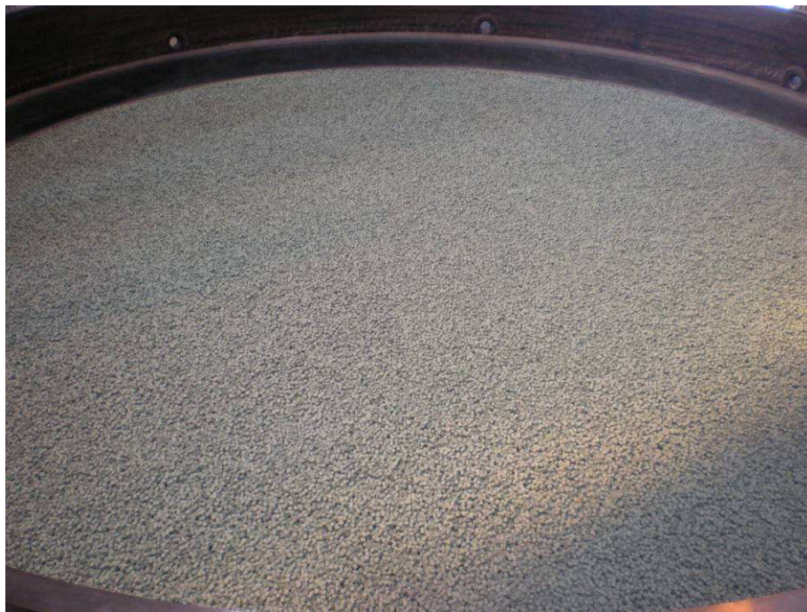
Figure 2: Installation of secondary catalyst in North burner
