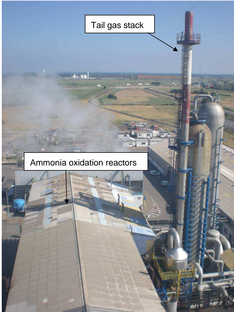
Figure 2: Close-up image of Montoir plant
