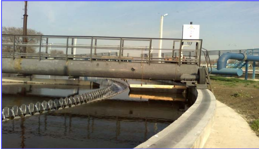
Fig.7. Sewage disposal plant were Heat Pump Station is planning to be install.
