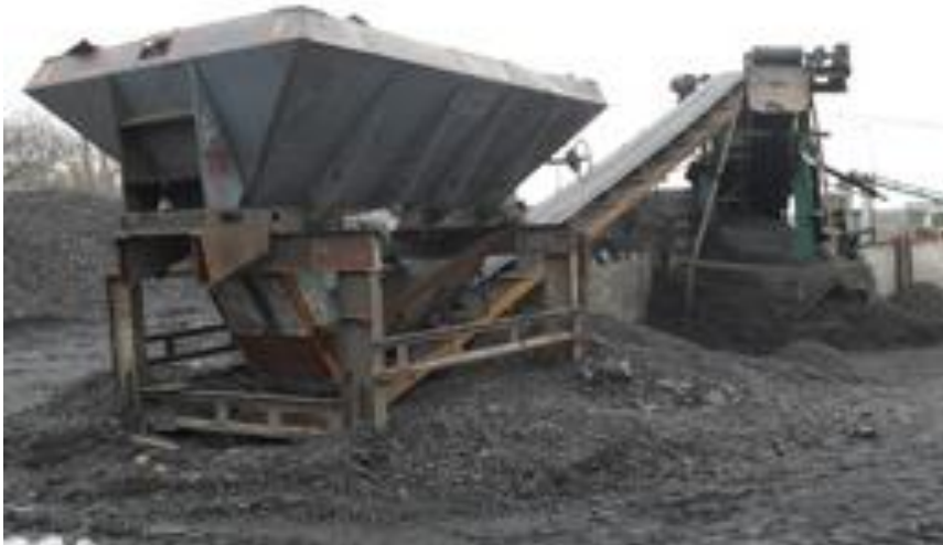
Fig.5 Bunker where rock mass is loaded.
