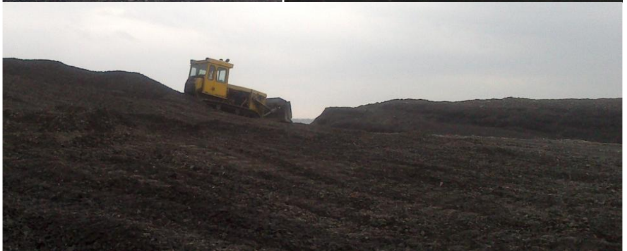
Figure 4 - Machinery involved in the project.
