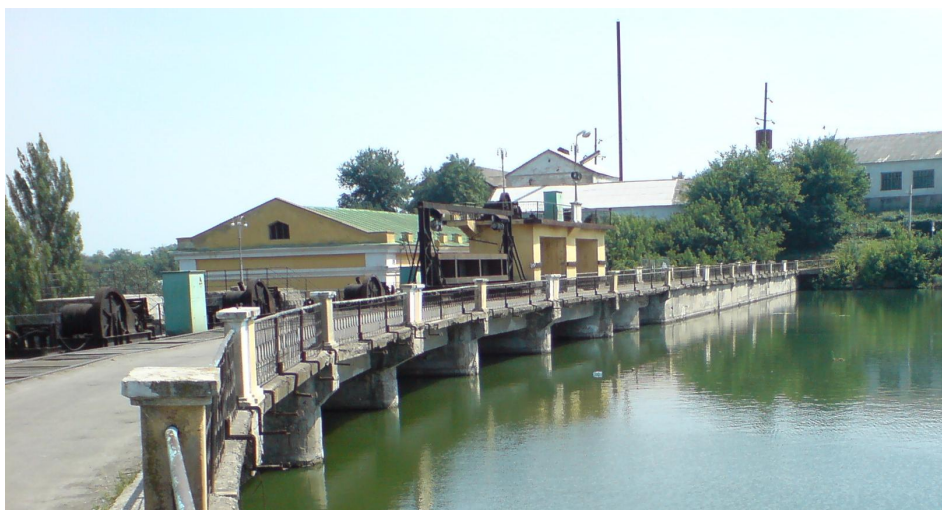
Fig. 5. Steblivska small HPP after renovation
