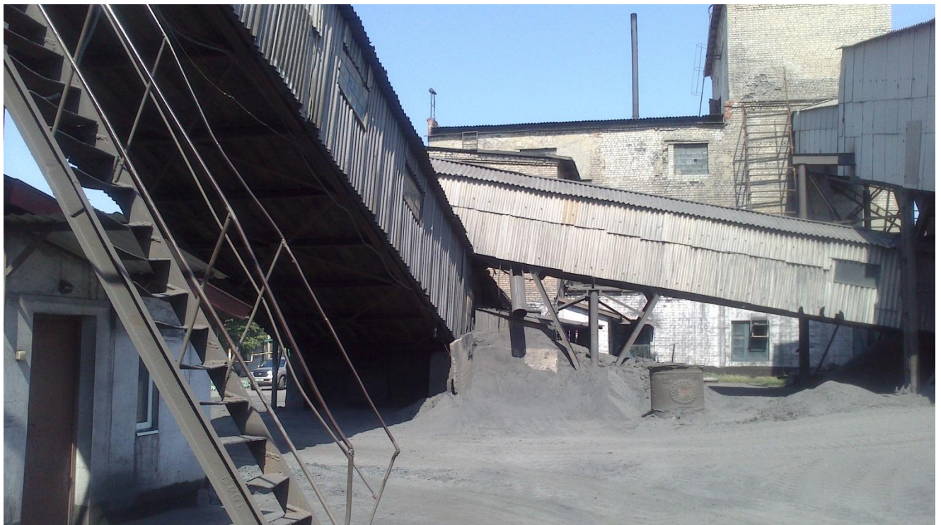
Figure 4 – Enrichment plant # 105 involved in the project.
