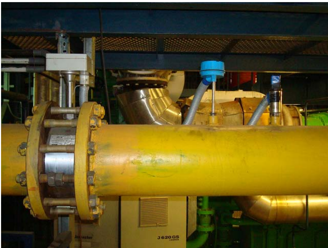
Figure 4: Sensors of flow, temperature and pressure at the CHP unit fuel methane pipeline In the table below the description of the secondary meters (indicated brown in the schema) are given:
