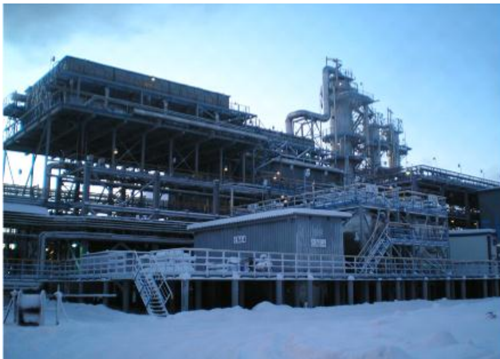
Fig. A.2-1. General view of the gas treatment plant
