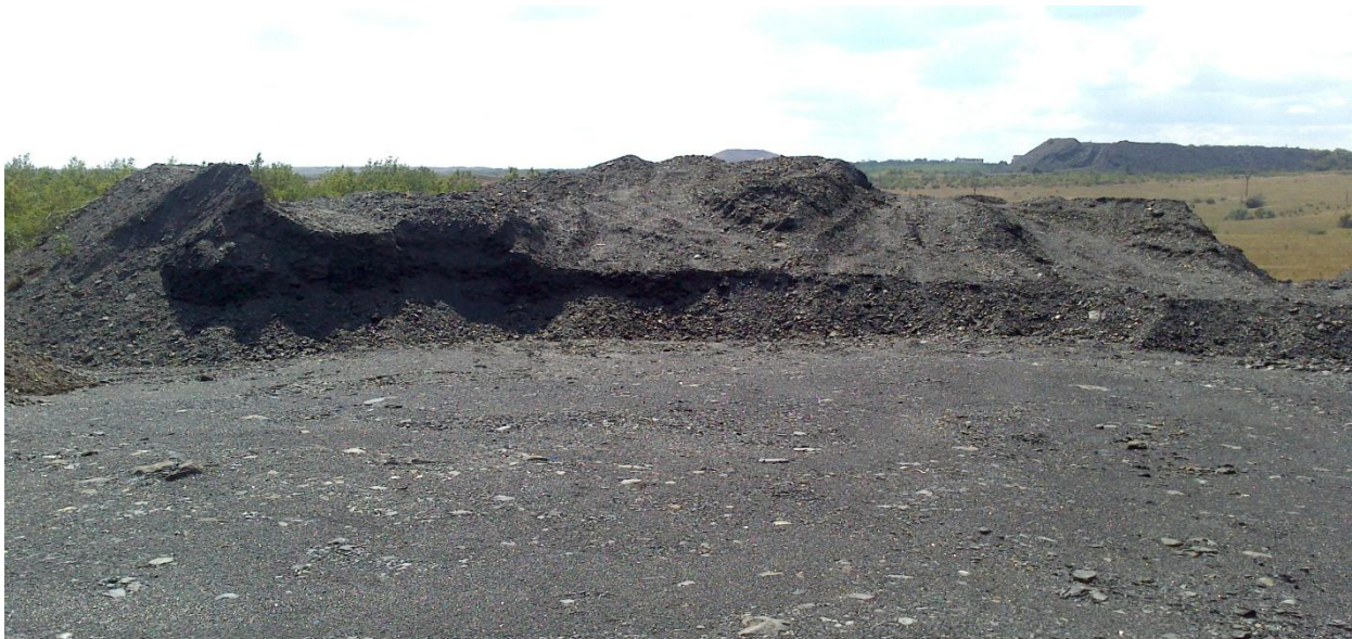
Figure 3 – The external appearance of the waste heap of former mine #18 under final dismantling stage.
