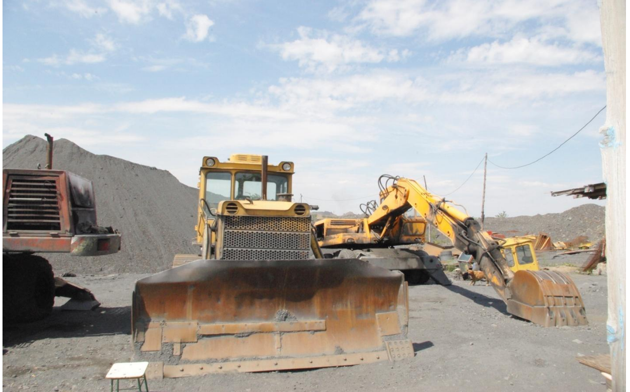
Figure 2 - The exterior of the waste heap under dismantling stage
