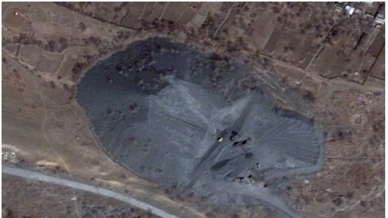
Figure 3 – The waste heap under dismantling stage, the appearance from the satellite
