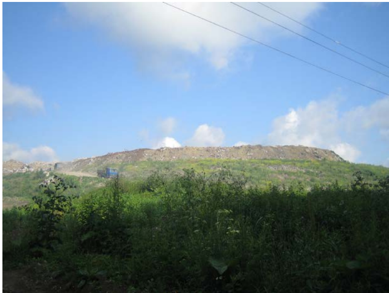
Figure A.4.1.4. Shirokorechenskiy landfill site
