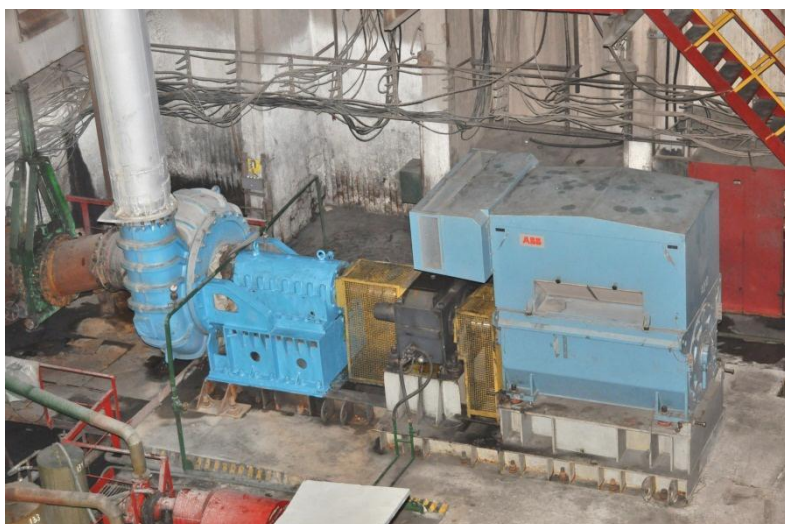
Figure 3 Dredging system HHD-49
